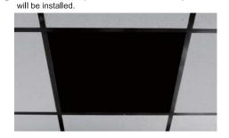
4. Carefully insert the LED Troffer Light into the removed ceiling.
