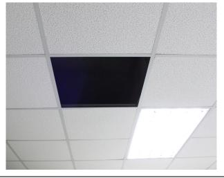
7. Remove the ceiling where the LED driver and the LED panel light will be installed.
